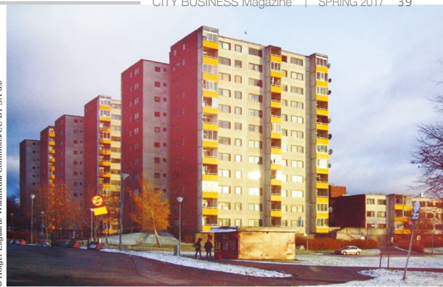
Flats from the Million Homes Programme of the 1950s-60s are now a regeneration challenge
